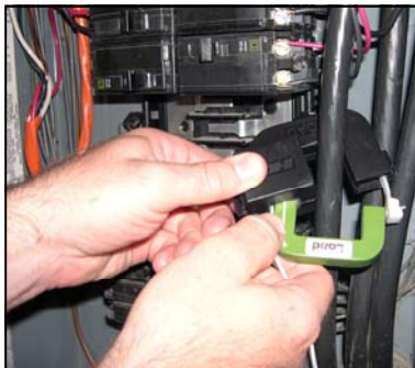
Fig. 1—Key advantage of electronic submeter is 0-2V split-core current sensor installed non-invasively around electrical feed being metered, which eliminates having to power down the load and makes for a quicker, safer and more profitable installation for the electrical contractor.
